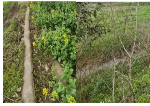
灌溉渠道现状
